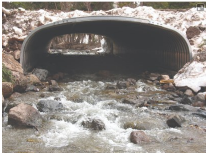
Figure 14: Example of a completed AOP culvert
